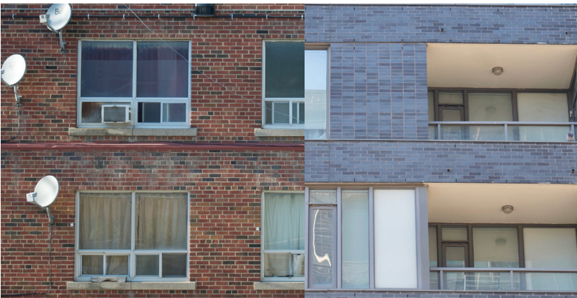
OLD AND NEW BUILDINGS
